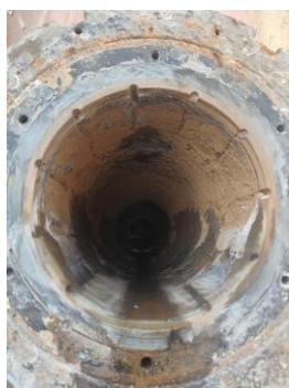
Figure 4. Vessel 7 (Lucky Star rice carrier) after 3 years: The cooling-water grooves were partially blocked by silt deposits due to silt buildup, diametral clearance 8.42 mm - exceeding the 6.0 mm allowable
