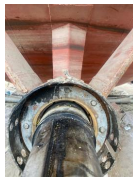
Figure 6. Vessel 9 (Hai Duong sand dredger) after 2 years: Bearing bore with delamination failure and embedded sand debris; shaft sleeve with deep longitudinal scratching and pitting
